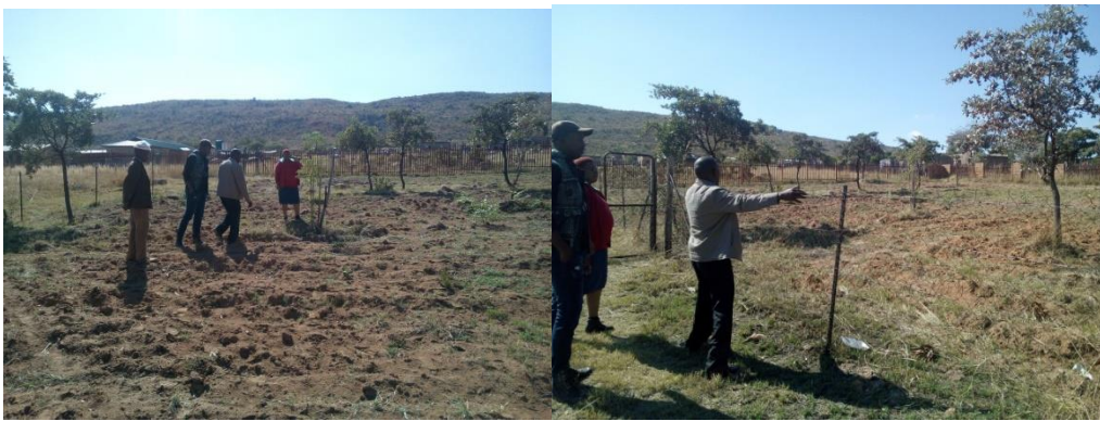
The fencing that needs repair to protect the site from livestock
